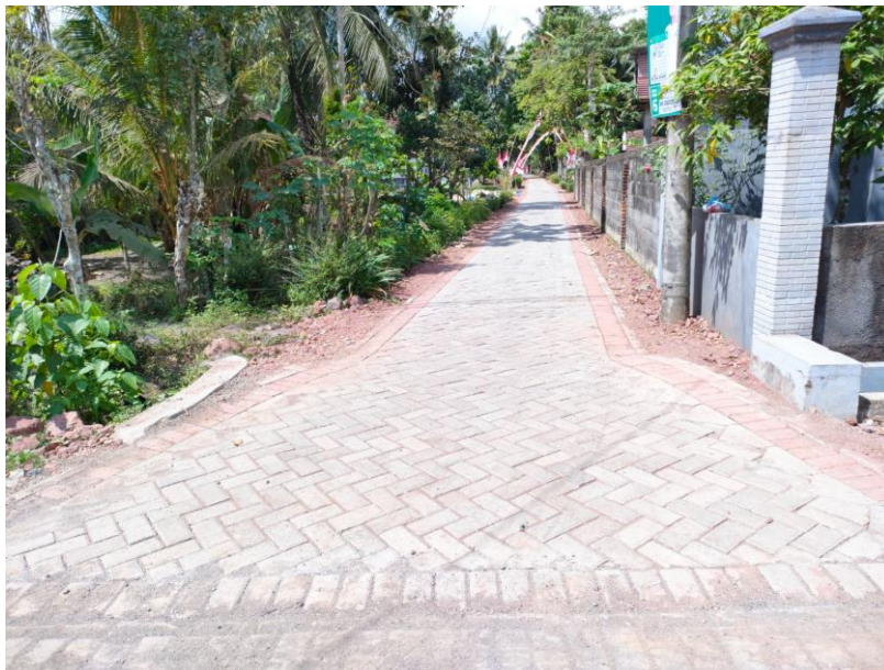
Gambar 4. Finishing Paving Blok
